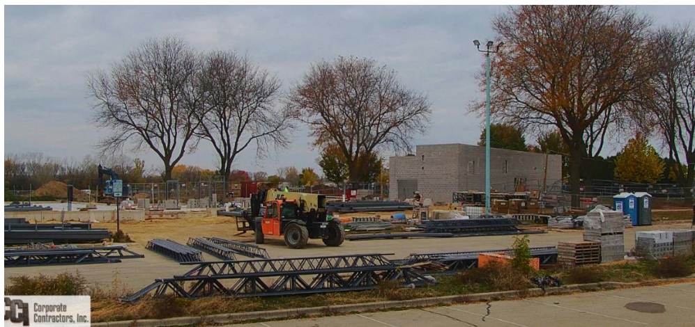
1 Steel on site at the Imagination Center. Photo credit: CCI.
