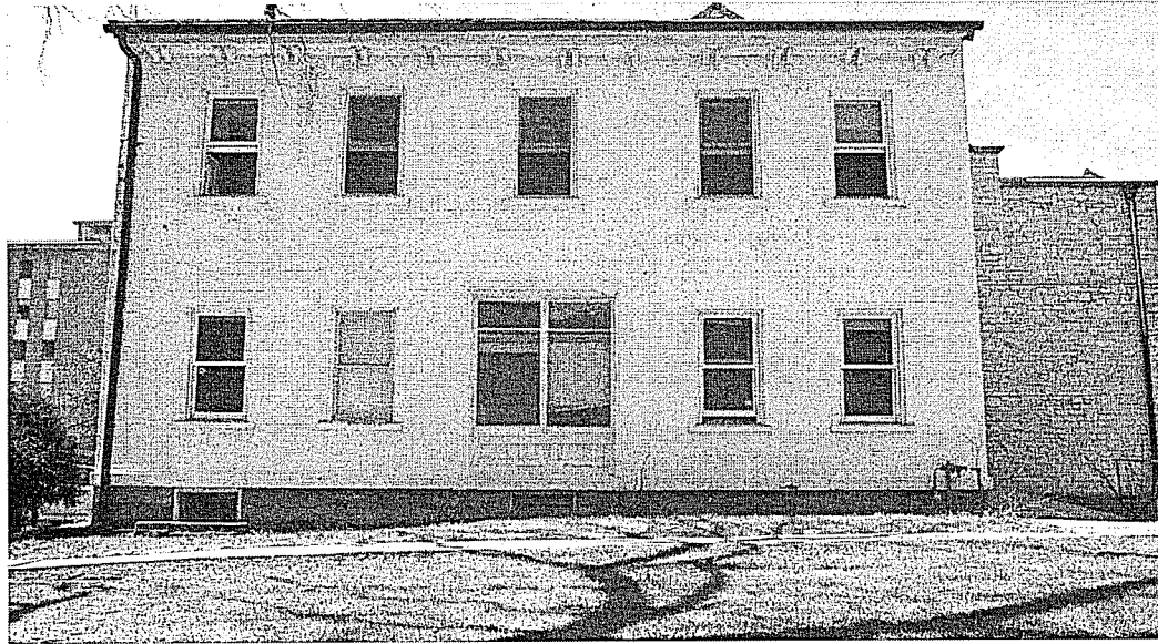
East Facade (historic main entry to residence)
