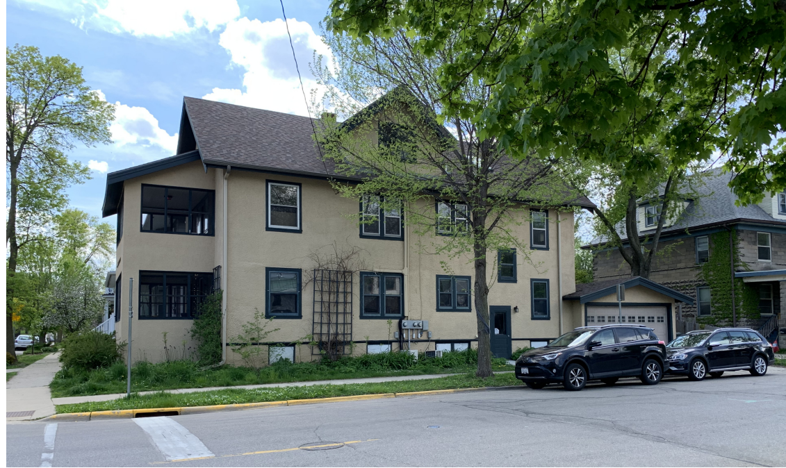
EXAMPLE OF NATURAL STUCCO EXTERIOR ON OPPOSITE CORNER OF BALDWIN AND SPAIGHT
