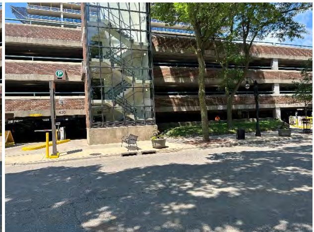
Frances Street (view across street)
