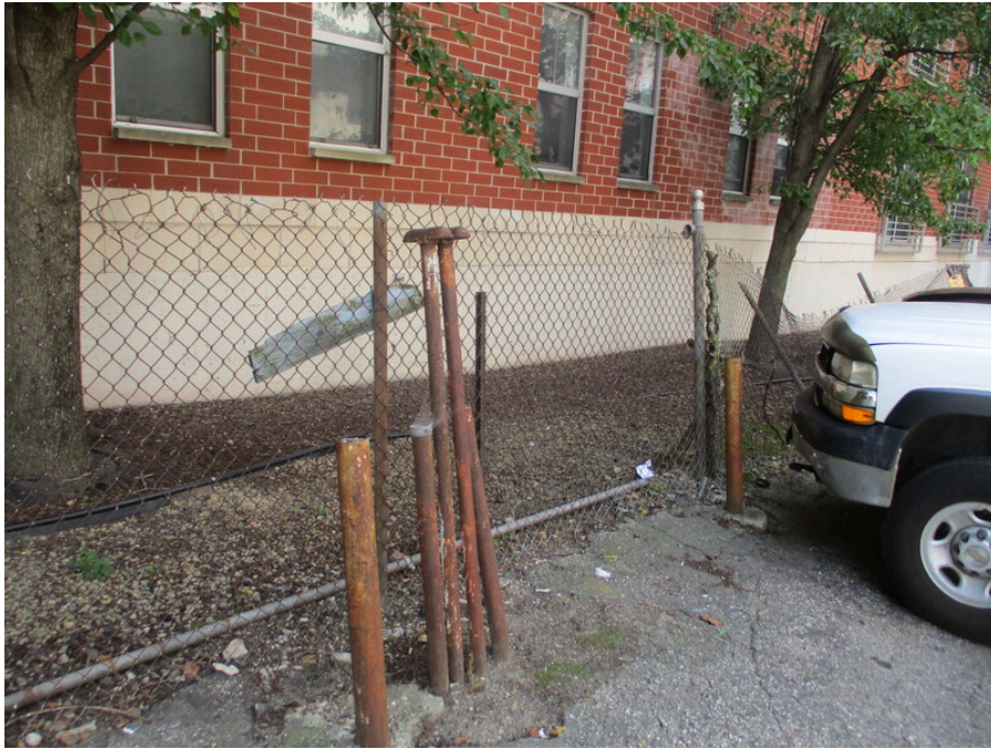
Photo 11: 415 W. Gilman Street-view fill and vent pipes, east side of property
