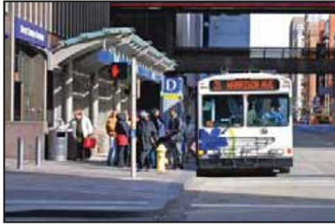
Bus Stop integrated into the building facade © 2006 Sitephocus, LLC., www.sitephocus.com
