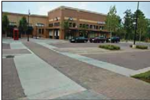
Raised or "tabled" crosswalks help make pedestrians more visible to motorists. A center island allows pedestrians to cross one direction of traffic at a time © 2006 Sitephocus, LLC., www.sitephocus.com
