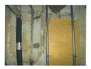
Photo is taken of basement foundation showing existing large cracks in limestone foundation wall that have been caulked. Existing piping has asbestos insulation covering original piping.
