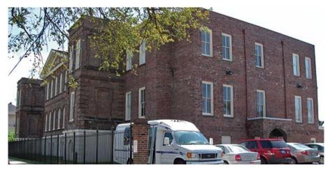
**Figure 9.** A simple, brick stair tower replaced two non-historic additions at the rear of this 1879 school building when it was rehabilitated as a women's and children's shelter. The addition is set back and it is not visible from the front of the school.
