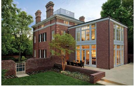
Figure 4. This glass and brick structure is a harmonious addition set back and connected to the rear of the Colonial Revival-style brick house. Cunningham/Quill Architects. Photos: © Maxwell MacKenzie.
