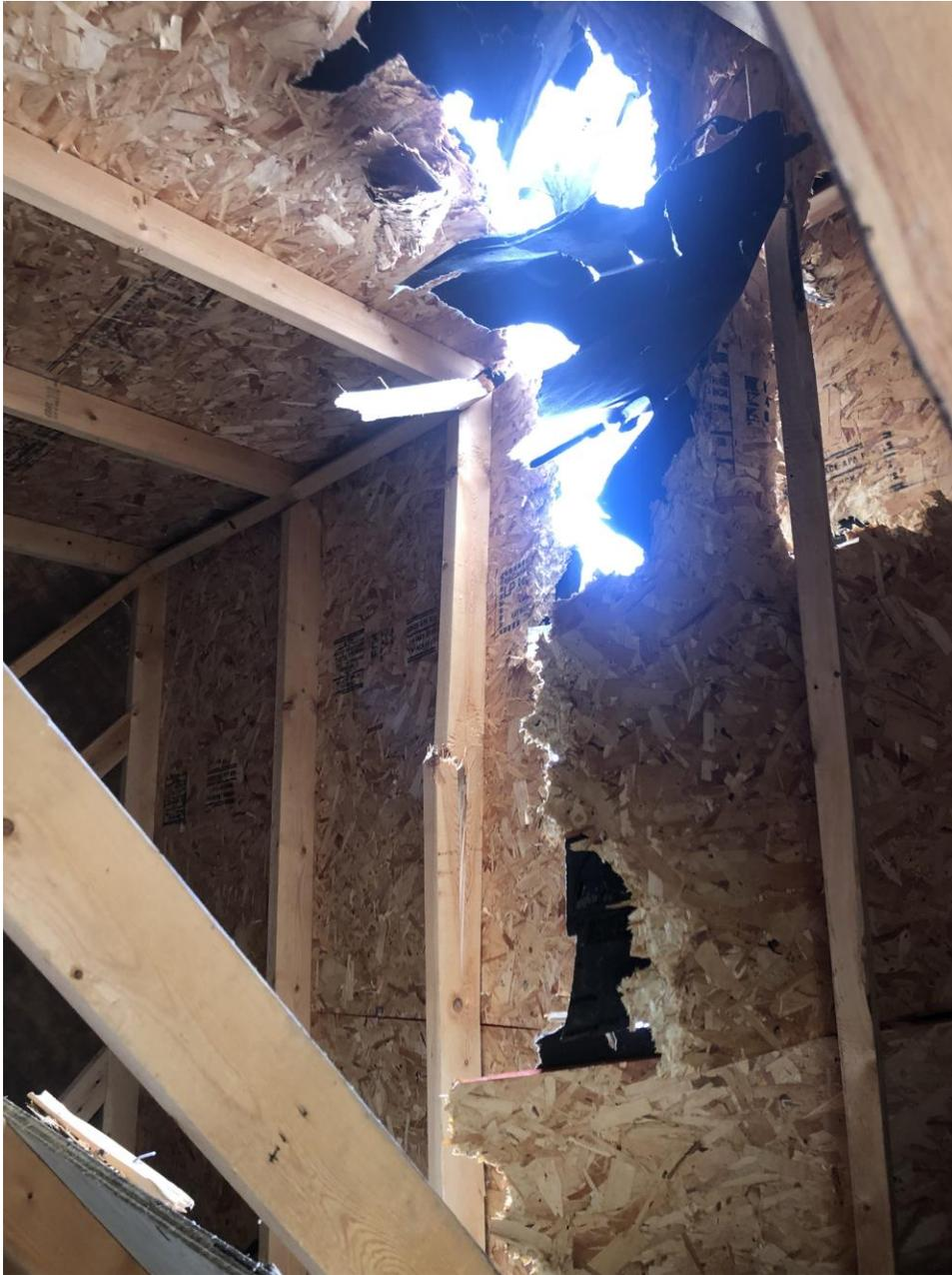
Interior photo of the damaged gable shed showing cracked wall and roof framing.
