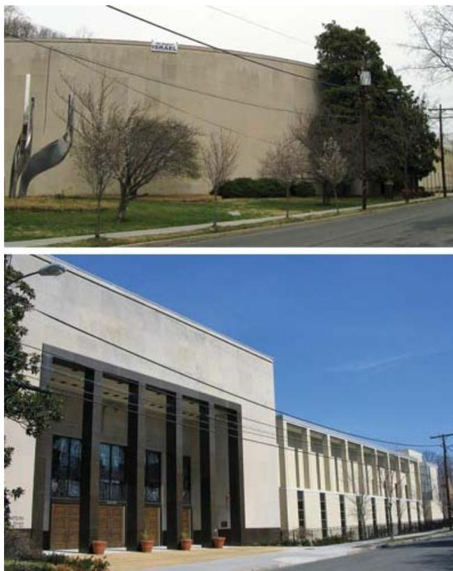
**Figure 12.** This 1954 synagogue (top) is accessed through a monumental entrance to the right. The new education wing (bottom) added to it features the same vertical elements and color and, even though it is quite large, its smaller scale and height ensure that it is secondary to the historic resource.
