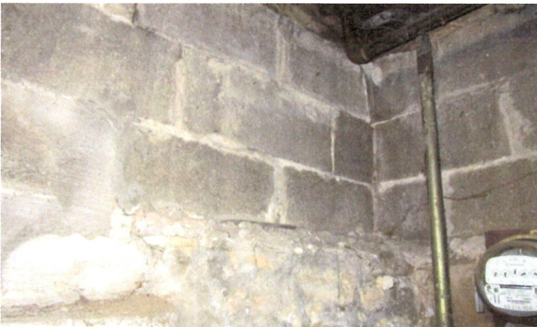
View of the original stone foundation walls topped with concrete block walls.
