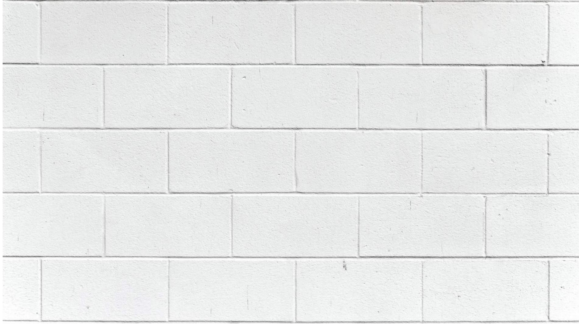
Existing CMU north and west wall. Cleaned, primed and painted to match board and batten metal panelsiding and roof
