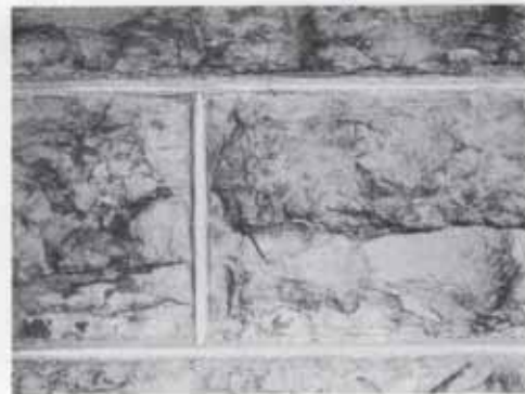
Figure 18. A cross-section of mortar joint types. (a) Grapevine joints on a mid-18th century brick building; (b) flush joints on a mid-to-late 19th century brick building; (c) beaded joints on a late-19th century brick building; (d) early-20th century beaded joints on rough-cut limestone where the vertical joints were struck prior to the horizontal joints; (e) raked joints on 1920s wire brick; (f) horizontal joints on a 1934 building designed by Frank Lloyd Wright were raked back from the face of the bricks, and the vertical joints were filled with a red-tinted mortar to emphasize the horizontality of the narrow bricks, and struck flush with the face of the bricks; (g) the joints on this 20th century glazed terracotta tile building are raked slightly, emphasizing the glazed block face. Photos: National Park Service Files (a,b,e); Robert C. Mack, FAIA (c,d,f,g).
