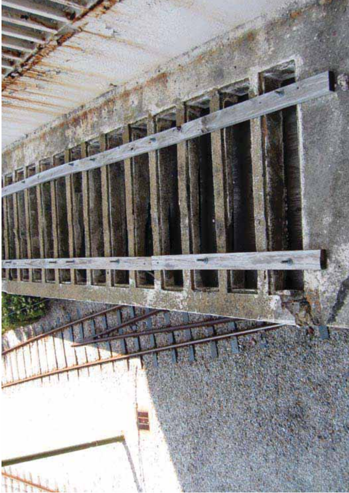
[5] Rebars in the reinforced concrete ceiling have rusted, causing the concrete to spall. The rebars must be cleaned of rust before the concrete can be patched. [6] Some areas of the concrete brise soleil screen on this building constructed in 1967 are badly deteriorated. If the screen cannot be repaired, it may be replaced in kind or with a composite substitute material with the same appearance as the concrete.
