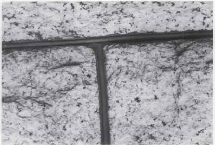
Figure 3. Good-quality repointing closely replicates the original in composition, texture, joint type and profile on this 19th century brick building (left), and on this late-19th century granite on H.H. Richardson's Glessner House in Chicago (right). Photos: Charles E. Fisher; Sharon C. Park, FAIA.
