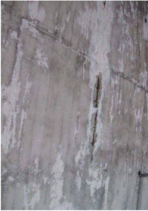
[5] Rebars in the reinforced concrete ceiling have rusted, causing the concrete to spall. The rebars must be cleaned of rust before the concrete can be patched. [6] Some areas of the concrete brise soleil screen on this building constructed in 1967 are badly deteriorated. If the screen cannot be repaired, it may be replaced in kind or with a composite substitute material with the same appearance as the concrete.
