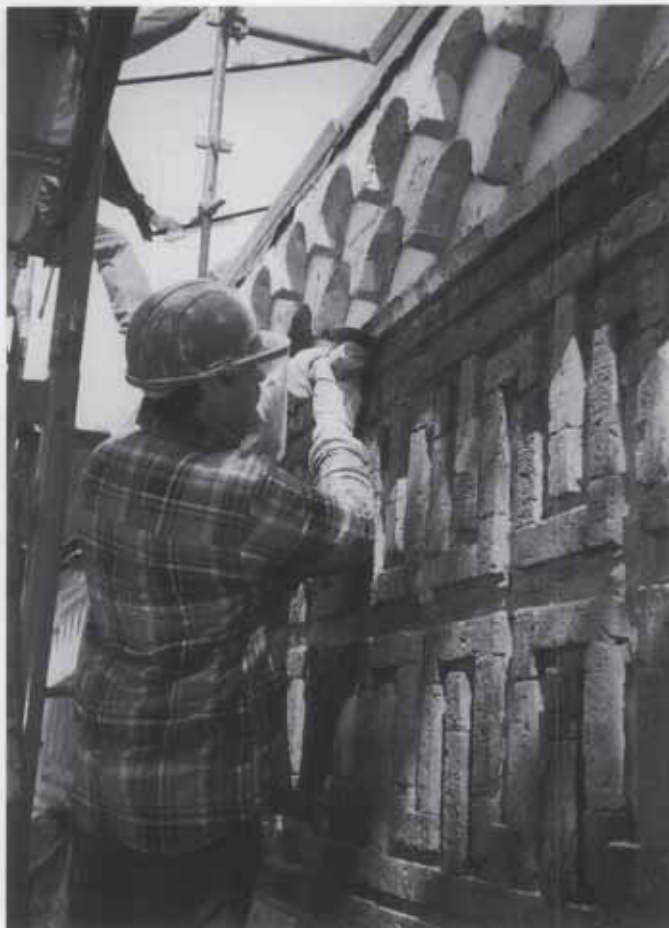
Figure 12.. A power grinder, operated correctly by a skilled mason may be used in preparation for repointing to cut wide, horizontal mortar joints, typical of many early-20th century brick structures without causing damage to the brick. Note the use of protective safety equipment. Photo: Robert C. Mack, FAIA.
