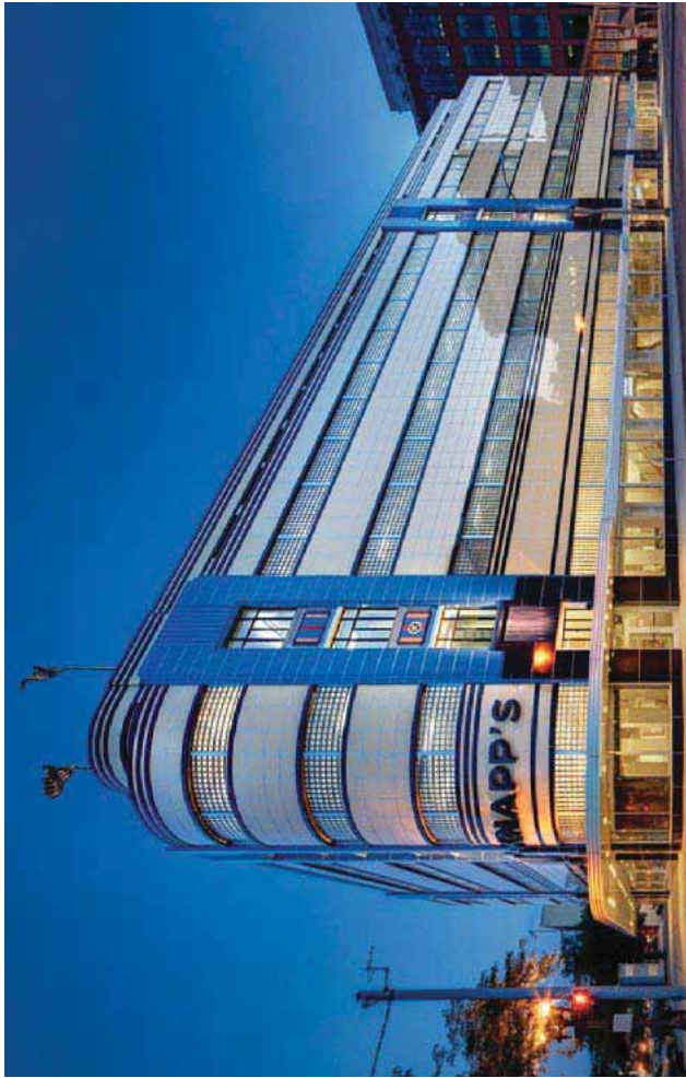
[7] (a) J.W. Knapp's Department Store, built 1937-38, in Lansing, MI, was constructed with a proprietary material named "Maul Macotta", made of enameled steel and cast-in-place concrete panels. Prior to its rehabilitation, a building inspection revealed that, due to a flaw in the original design and construction, the material was deteriorated beyond repair. The architects for the rehabilitation project devised a replacement system (b) consisting of enameled aluminum panels that matched the original colors (c). Photos and drawing (a-b): Quinn Evans Architects; Photo (c): James Haefner Photography.
