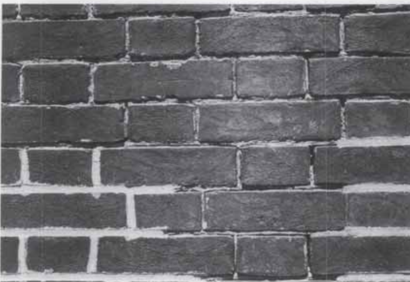
Figure 4. (left) The poor quality of this repointing—it appears to have been “tooled” with the mason’s finger—does not match the delicacy of the original beaded joint on this 19th-century brick wall. (right) It is obvious that the repointing on this “test patch” is not an appropriate replacement mortar joint for this early-19th century stone foundation. Photos: Lee H. Nelson, FAIA.
