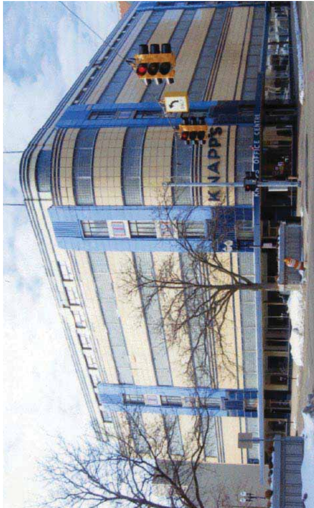
[7] (a) J.W. Knapp's Department Store, built 1937-38, in Lansing, MI, was constructed with a proprietary material named "Maul Macotta", made of enameled steel and cast-in-place concrete panels. Prior to its rehabilitation, a building inspection revealed that, due to a flaw in the original design and construction, the material was deteriorated beyond repair. The architects for the rehabilitation project devised a replacement system (b) consisting of enameled aluminum panels that matched the original colors (c). Photos and drawing (a-b): Quinn Evans Architects; Photo (c): James Haefner Photography.
