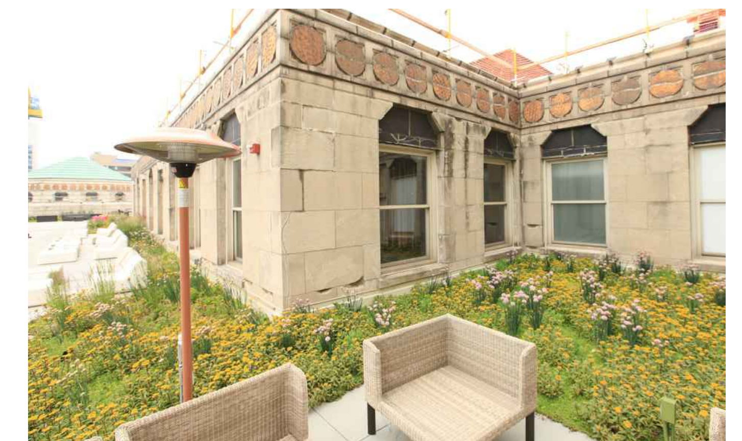
GREEN ROOF OUTDOOR RESIDENTIAL TERRACE
