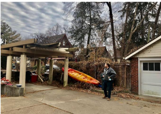
CARPORT ADDED IN THE 80'S. THE ROOF IS CANVAS AND THE WOOD STRUCTURE IS ROTTED BEYOND REPAIR AND WOULD REQUIRE CONSTRUCTION. CONCRETE COLUMNS IMPEDE CAR-DOOR CLEARANCE. LOCATION OF THIS CAR PORT RESTRICTS PEDESTRIAN ACCESS TO THE BACK DOOR ENTRY OF THE HOUSE.
