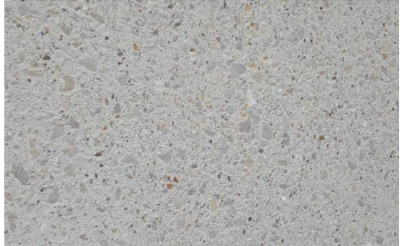
SAND BLASTED TILT-UP CONCRETE WALL
