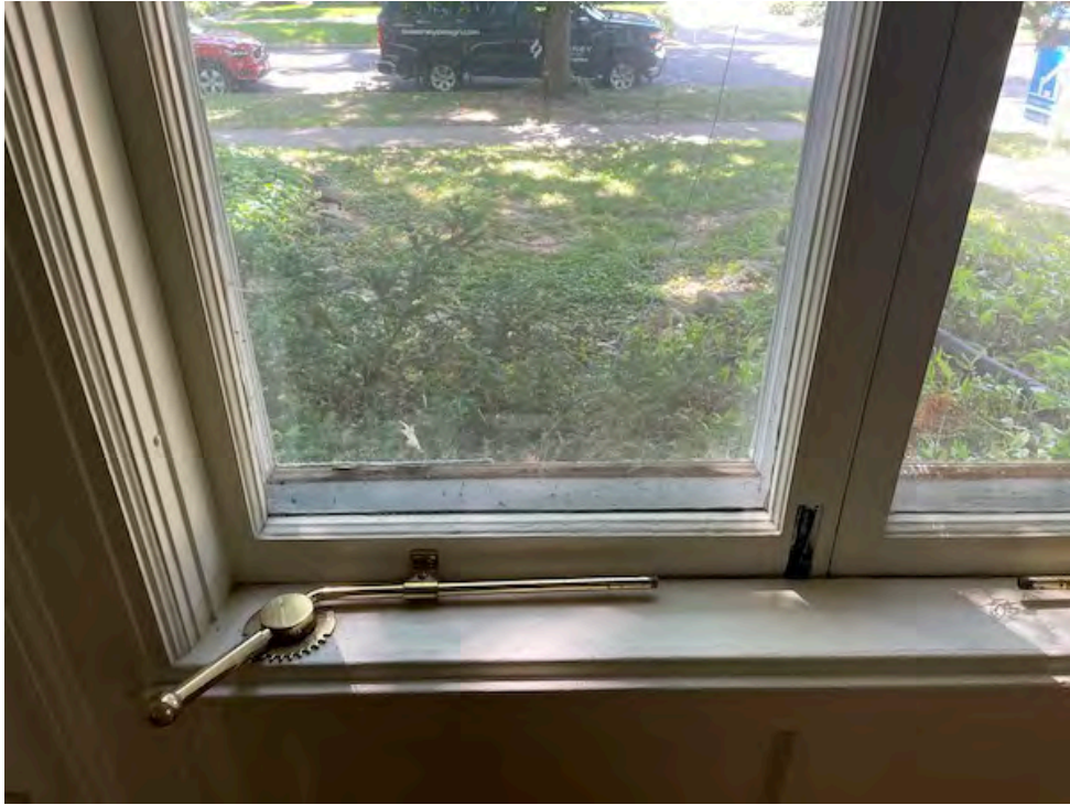
Casement window on main level
