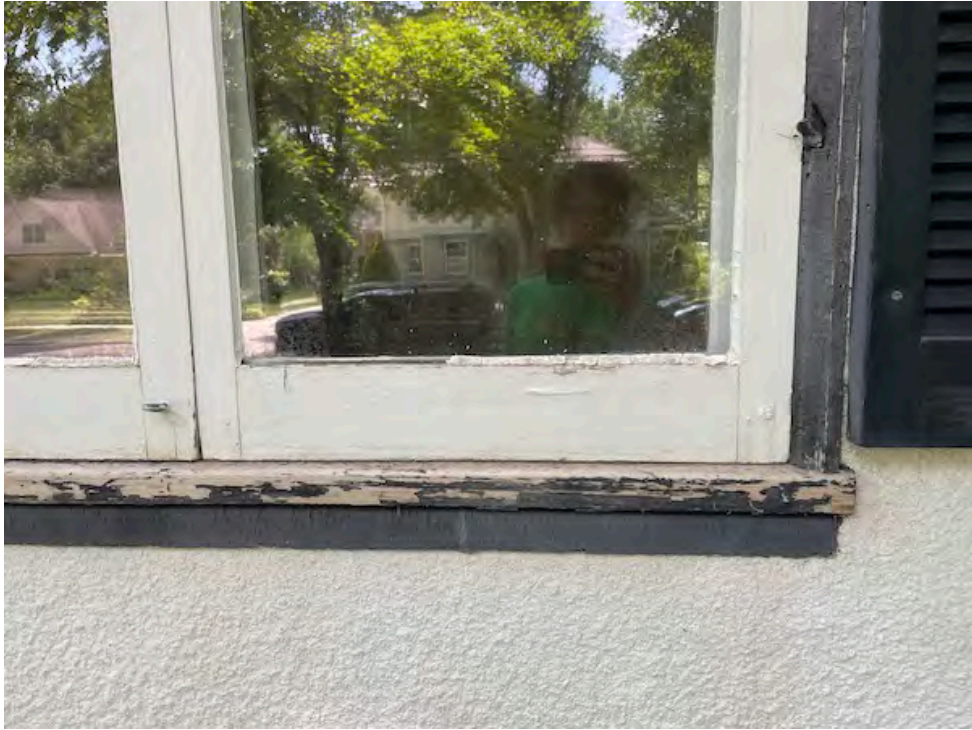
Exterior trim & storm
