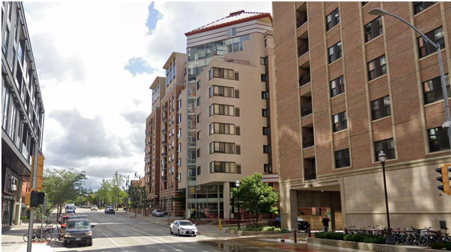
LOOKING NORTH / EAST DOWN W. GORHAM ST.
