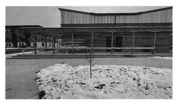
A temporary wood railing has been installed to restrict access to the stairway portions having nonuniform riser heights as a condition of occupancy.
