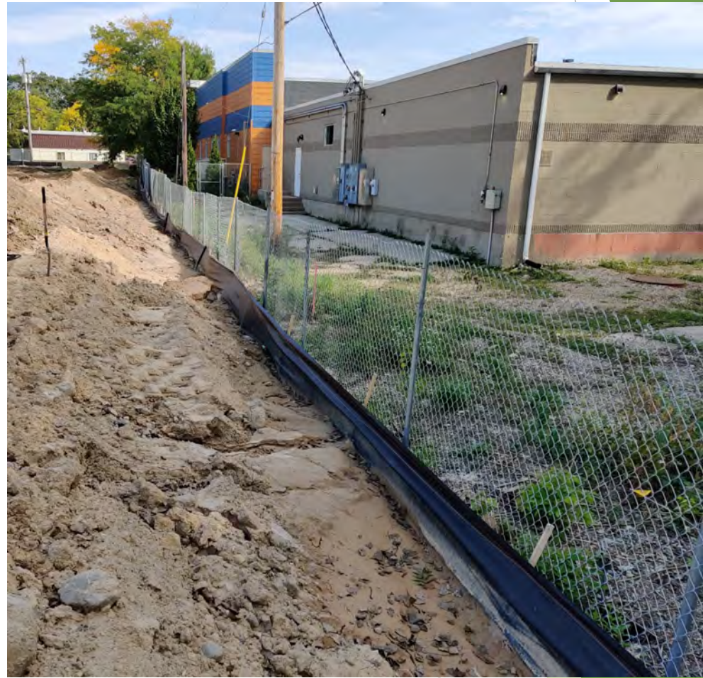
Cedar Street Silt Fence
