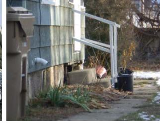
front walk cracked and sunken; retaining wall shifting with pieces missing; driveway uneven and chunks missing; fence leaning; sunken steps safety hazard
